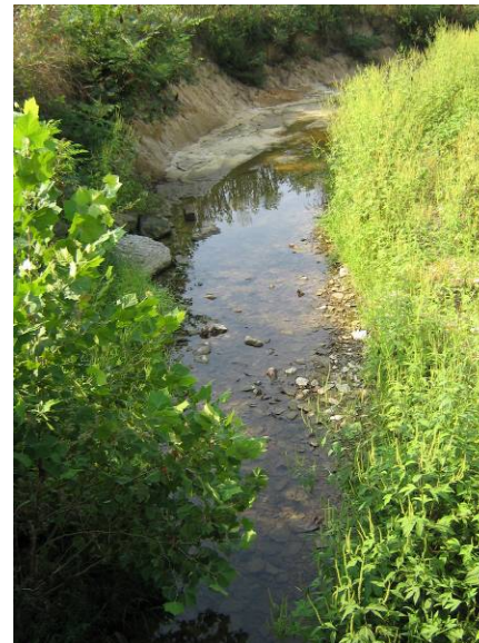
Downstream. Note erosion on bank in background.
